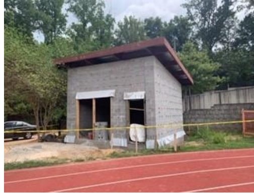
CSK- Storage metal deck installation
