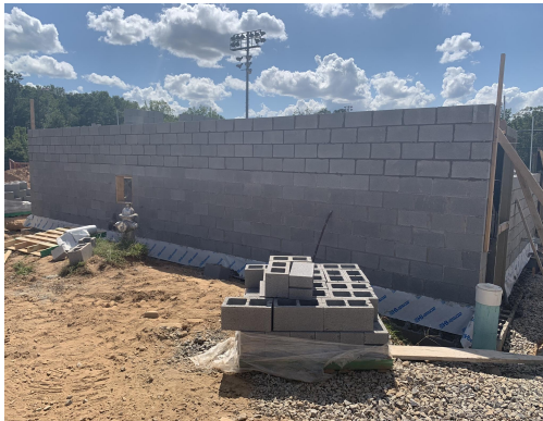
CSK- Concession CMU wall installation
