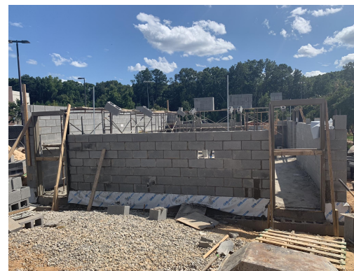
CSK- Concession exterior door frame installation
