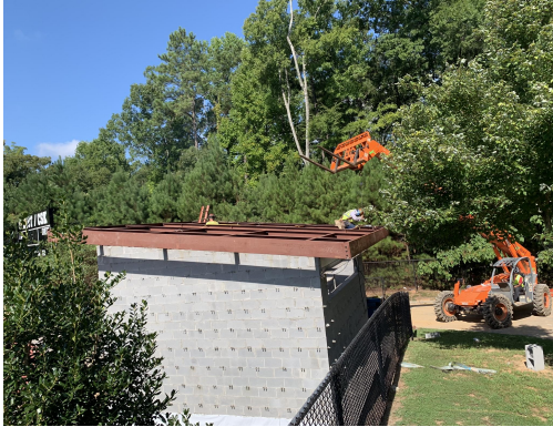
CSK- Storage steel installation
